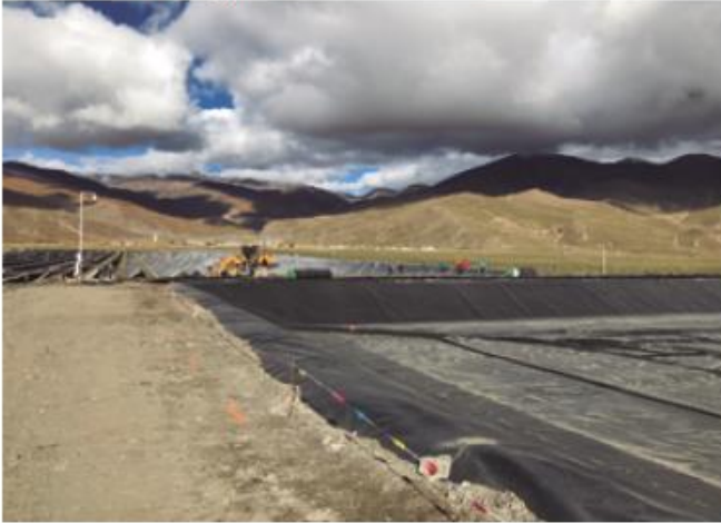
1. Dig a hole in the ground and put the soil around the edges.
